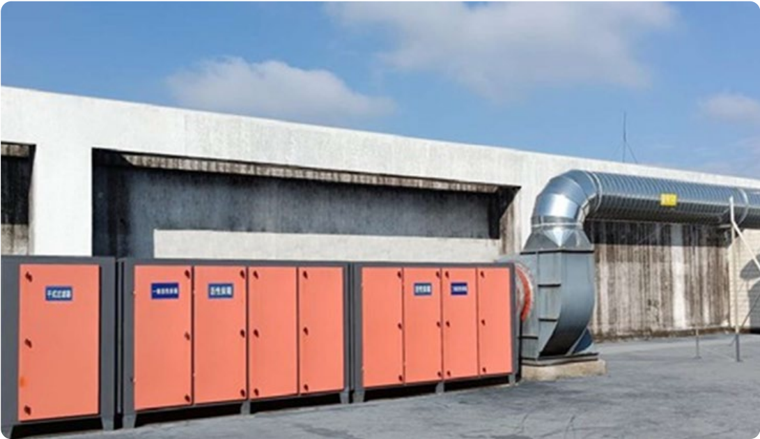
Production Exhaust Smoke Purification Facilities
